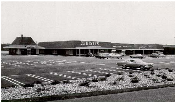
Mashpee Commons Before: Retail strip mall with retail and professional office; illustrates the domination of the automobile
