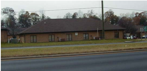
Improper orientation – Buildings should not orient a secondary façade with mechanical equipment facing the primary street
