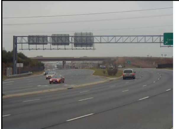
Prince William Parkway, looking west toward Horner Road Bridge
