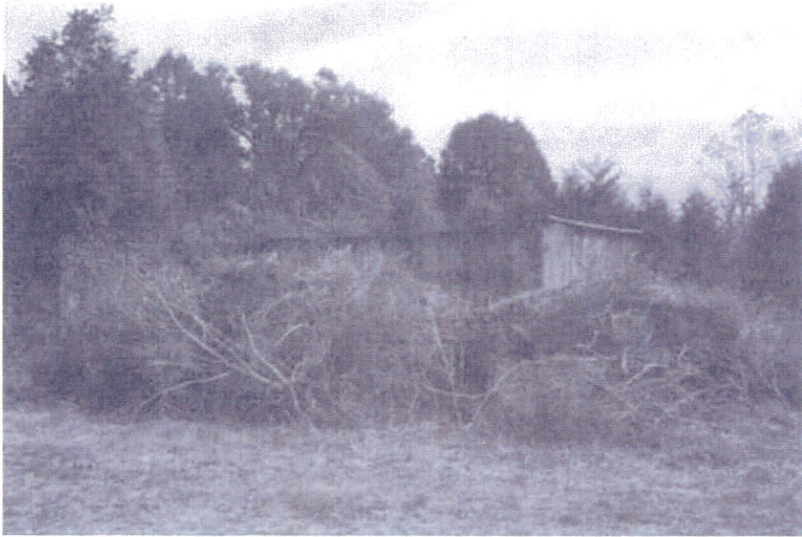
11. Exterior, Shed Roof Storage Shed, Southwest Property Boundary
